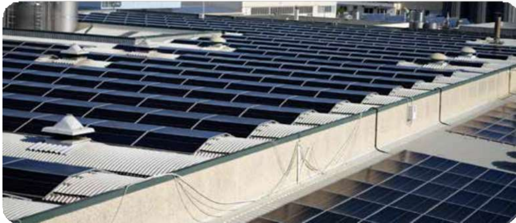
SYSTEMS FOR INDUSTRIAL ROOFS 799 kWp system with TILT system
