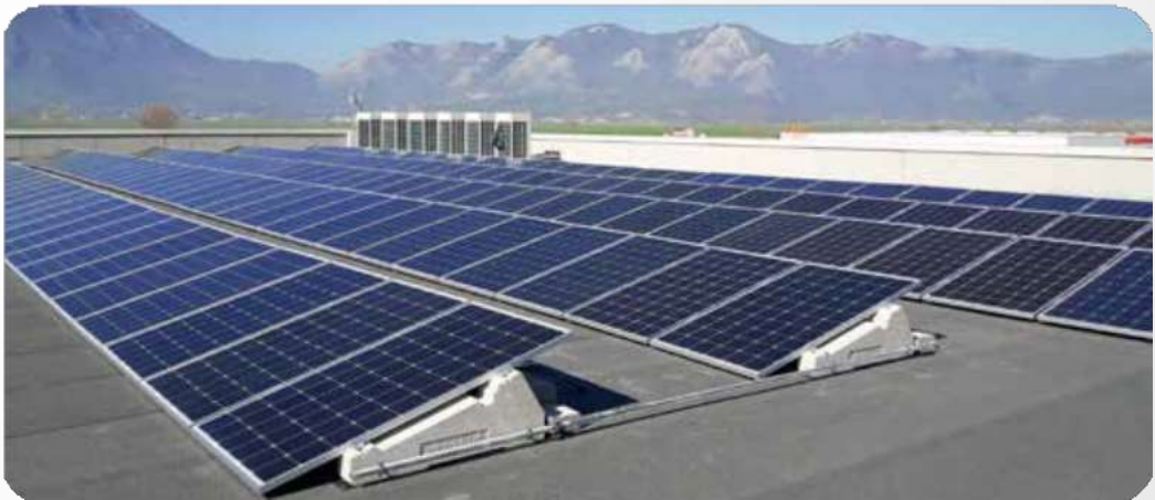
FLAT ROOF SYSTEMS 50 kWp system built with 15° ballast system - ZC1564
