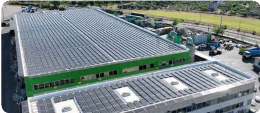
LOW-LOAD SYSTEMS FOR FLAT ROOFS 1.2 MW system built with SPIDERNET support and sunshade system
