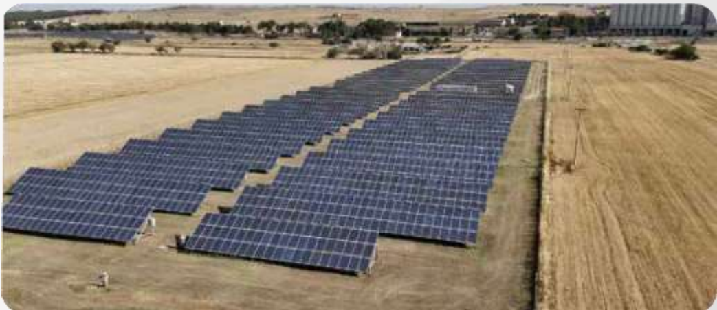
SYSTEMS FOR PHOTOVOLTAIC PARKS 800 kW plant built with INTERRA BIPALO structure
